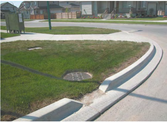
Figure X. East Clayton project first phase street drain systems. Conventional storm drain inlets on streets have been eliminated. Instead rainwater is directed through slotted curb to grassy boulevard, where it can infiltrate and enter infiltration basin under drain inlet. Amounts in excess of infiltration capacity of basin are directed to conventional storm drain pipes to storm drain ponds and then to stream.
