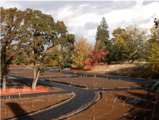
Figure X. Foreground streets are rear lanes for the future Pringle Creek development. Thirteen foot wide fire access lane is paved with pervious asphalt bordered by crushed stone infiltration verges. Filter fabric visible at edges contains the crushed stone base preventing migration of soil fines into the reservoir.
