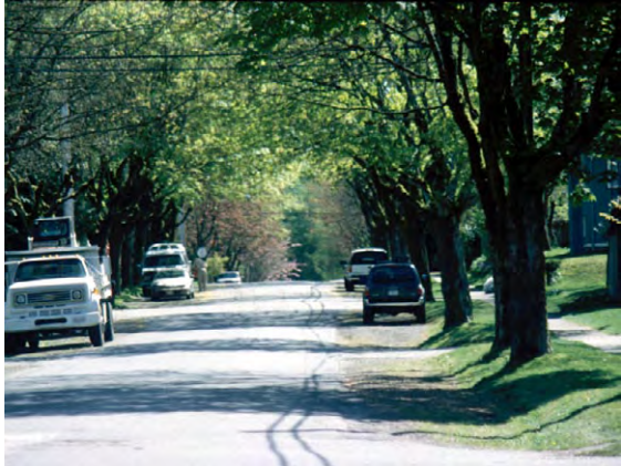
Figure X. Blenham Street, Vancouver, B.C. This street is characteristic of most streets built in the city prior to 1950. Two 7' wide crushed stone paved parking strips astride a 14' two way travel way for a total "curb to curb" width of 28'. Note grading of tree boulevard which effectively prevents cars from migrating onto soft shoulder. Sidewalks are included on both sides, one of which is visible to the right. Total ROW width is 60'.
