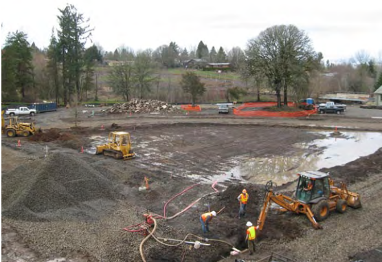
Figure X. The standing water seen here is actually the high water table revealed during the winter. The finished road surface is only a few inches above this point yet stays dry as water travels through the street section and surrounding soils via interflow, emerging in the banks of pringle creek almost visible in the distance beside the trees. The surface of the creek is only a foot or two lower than the water table, but sufficient to draw down the water if interflow is not impeded.
