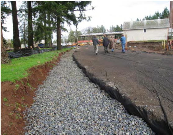
Figure X. The pervious paving used at the Pringle Creek Sustainable Community in Salem, Oregon uses crushed basalt aggregates as a structural base which also acts as water storage.
