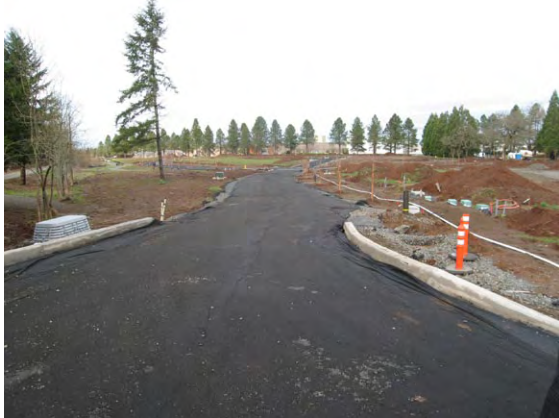
Figure X. Construction sites are dirty places, and dirt can quickly destroy investments in pervious pavements. At the Pringle Creek project streets were covered with filter fabric, as can be seen in this photograph, until the most disruptive phases of the site construction were complete.
