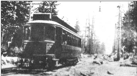
Figure X. Fourth Avenue Streetcar line freshly installed. Streetcars were provided before roads were improved or land subdivided for homes as a necessary precondition for development. Here is the scene a few years before these other urban features are built. Source: Vancouver: The Way it Was (Whitecap books)
