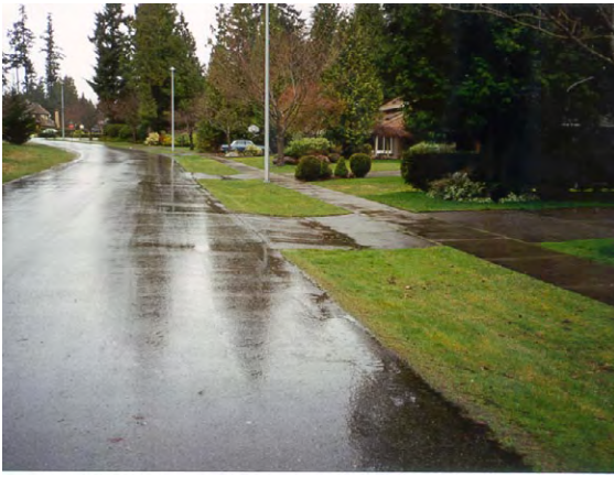
Figure X. Amble Greene project, Surrey BC. Curbless streets allow rain water to flow unimpeded along the entire length into lowered boulevard. Infiltration for most storms occurs in the wide boulevard, enhanced by invisible infiltration galleries below.
