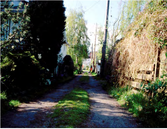
Figure X. Traditional Vancouver, BC lane paved with crushed stone. Areas outside of tire tracks have grown over creating healthy root zones for plant growth and associated infiltration.
